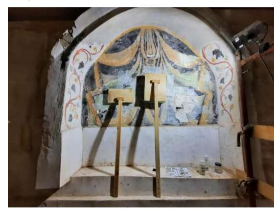
Support system set up before grouting
