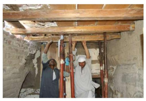
Taking out rotten beams in the antechamber by sliding them sideways (2019)
