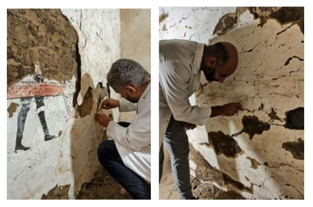
Securing mud plaster by rendering the edges, western walls on ground floor
